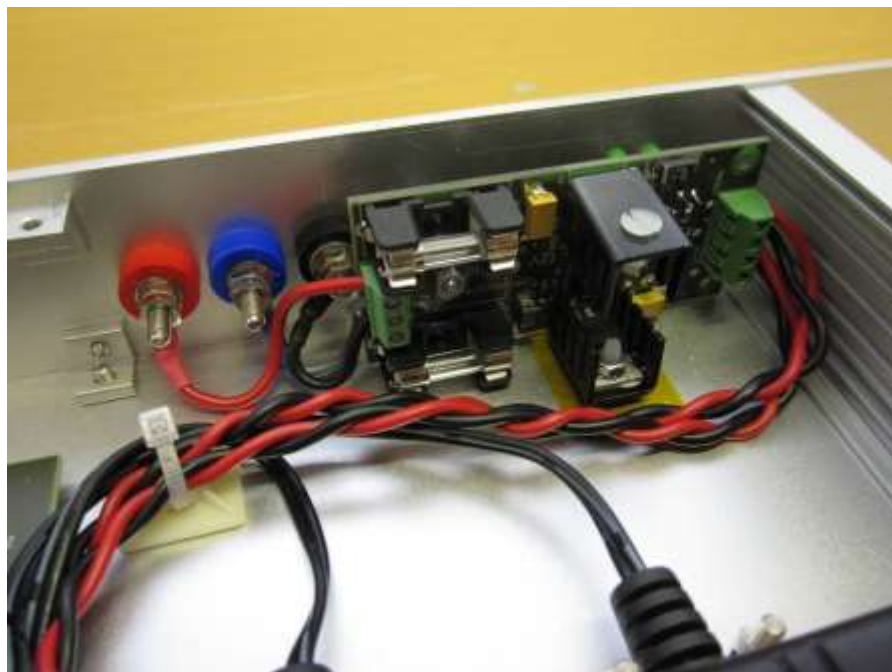
Figure 6: Voltage regulator unit with fuses. If there is no voltage at the regulator output but the leds are on (and regulator switch is on), check the fuses.
